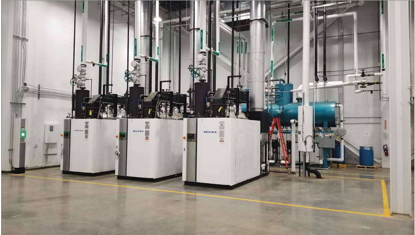
FIGURE 1. Miura's modular, once-through, watertube design boasts the ability to rapidly generate full steam, even from a cold start (on-demand steam).
