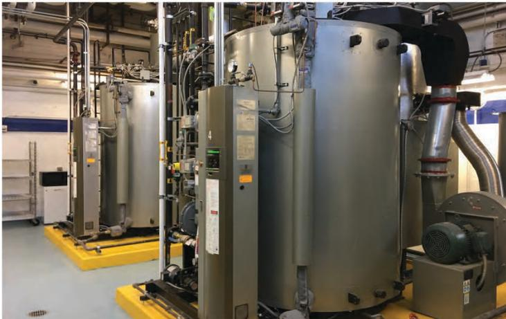
The 'floating header' concept allows for even thermal expansion of the tubes, therefore reducing stress points within the boiler." The 'leaky tube' problems associated with firetube and bent watertube designs have been eliminated.
