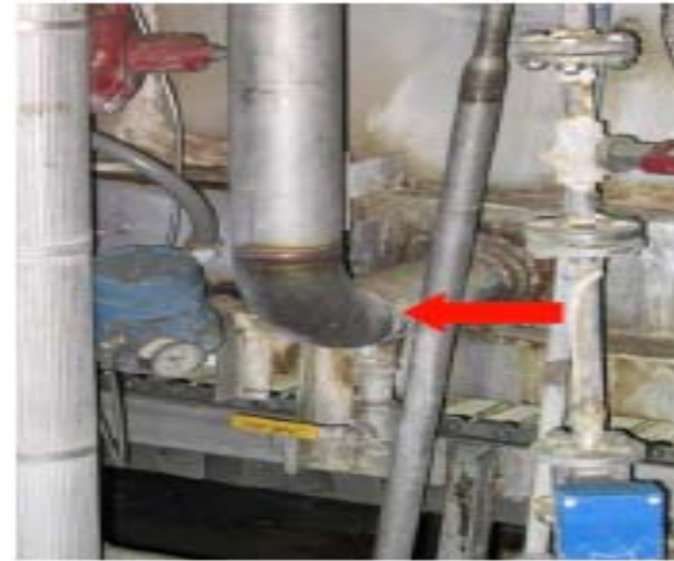
Rice Steam supply w/ no trap, separator or filter
